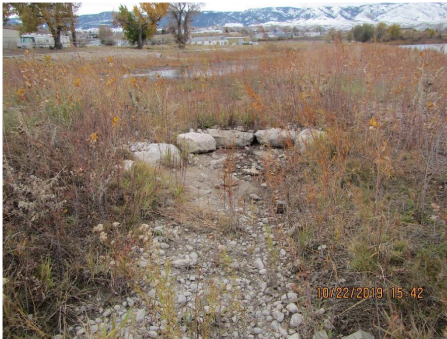
FIGURE A.5.24. Site 2 & 3 - Wyoming Blvd, at downstream set of wetland cross vanes, looking up at cross vane 40.
