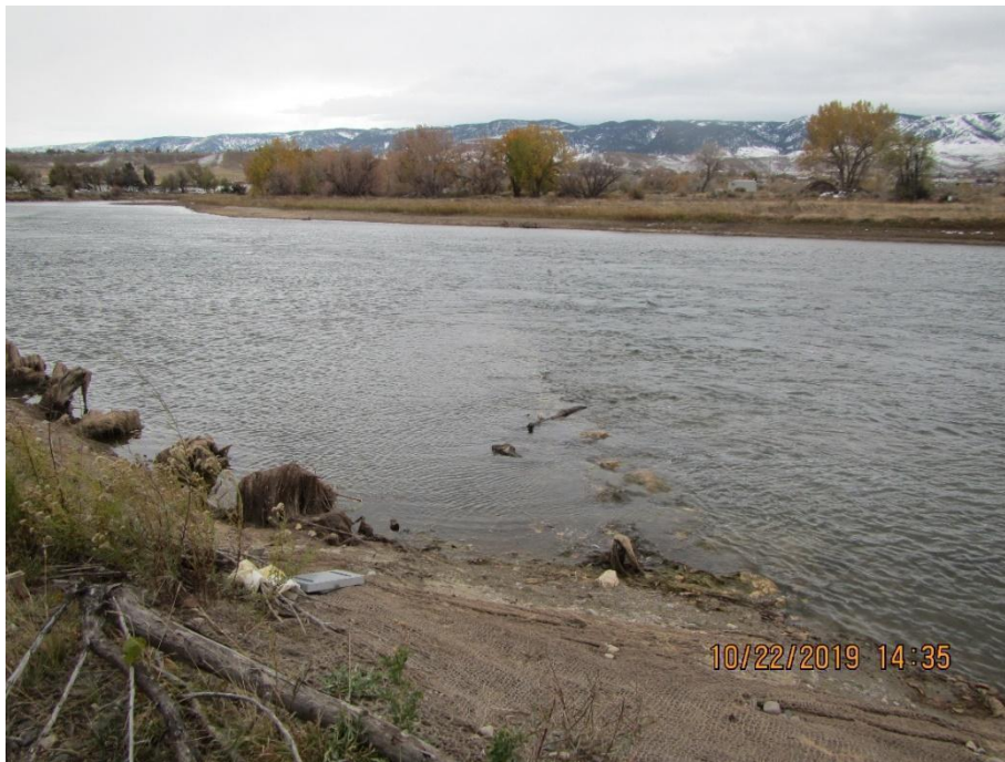
FIGURE A.5.14. Site 2 & 3 - Wyoming Blvd, standing at rock vane 4 on river right, looking slightly upstream, in direction of rock vane 4. Boulders in the vane are visible near the bank.
