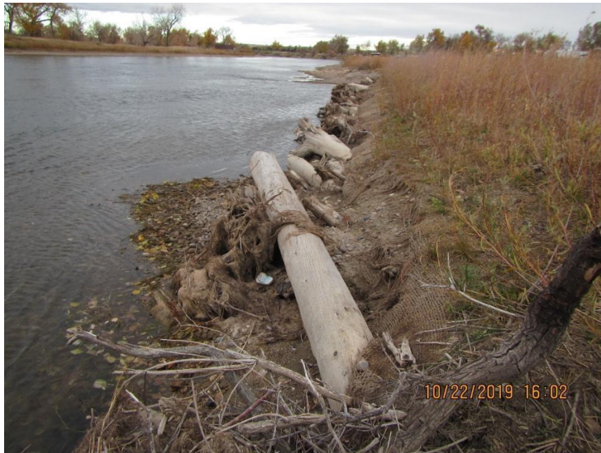
FIGURE A.5.3. Site 2 & 3 - Wyoming Blvd, standing upstream of toe wood 2, looking downstream.
