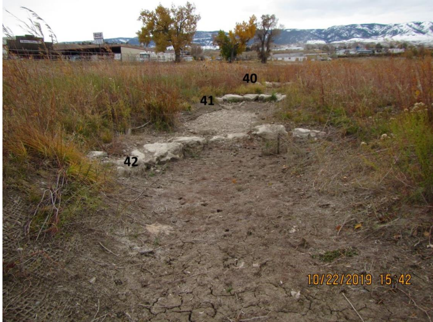
FIGURE A.5.23. Site 2 & 3 - Wyoming Blvd, at downstream set of wetland cross vanes, looking up at cross vanes 40,41, and 42.
