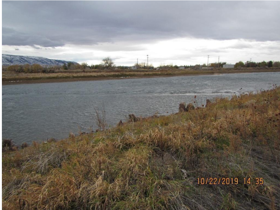
FIGURE A.5.15. Site 2 & 3 - Wyoming Blvd, standing just upstream of rock vane 4 on river right, looking slightly downstream, in direction of rock vane 4. The vane's influence on streamflow is visible at these flows past the channel center.
