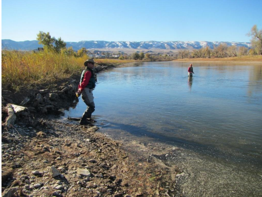
FIGURE A.5.13. Site 2 & 3 - Wyoming Blvd, standing just downstream of rock vane 3 on river right, looking upstream at rock vane 2. The two individuals are standing on the first and last visible boulders of rock vane 3. This photo is from October 2018, as the boulders could not be located in 2019.
