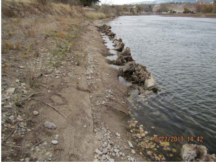
FIGURE A.5.7. Site 2 & 3 - Wyoming Blvd, standing at middle of toe wood 4, looking upstream at upper half of toe wood 4.
