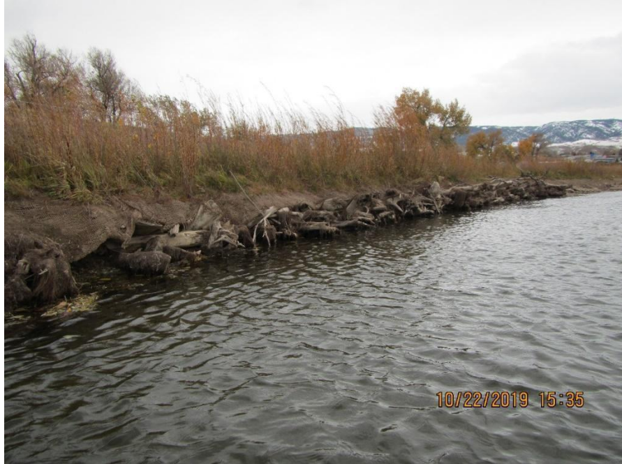
FIGURE A.5.5. Site 2 & 3 - Wyoming Blvd, at middle of toe wood 3 in-stream, looking at upstream half of toe wood 3.
