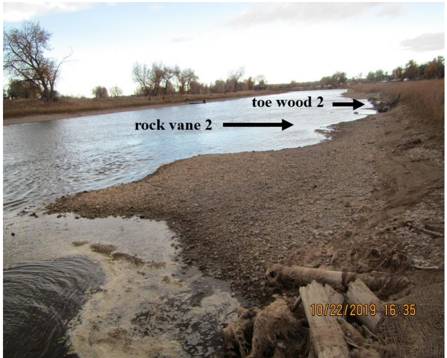
FIGURE A.5.12. Site 2 & 3 - Wyoming Blvd, standing just upstream of rock vane 2 on river right, looking downstream at rock vane 2 (rocks not visible in photo).
