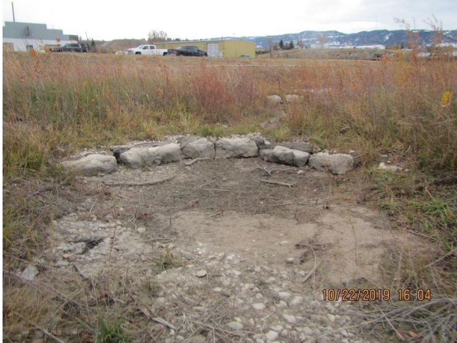
FIGURE A.5.21. Site 2 & 3 - Wyoming Blvd, at upstream set of wetland cross vanes, looking at cross vane 38.
