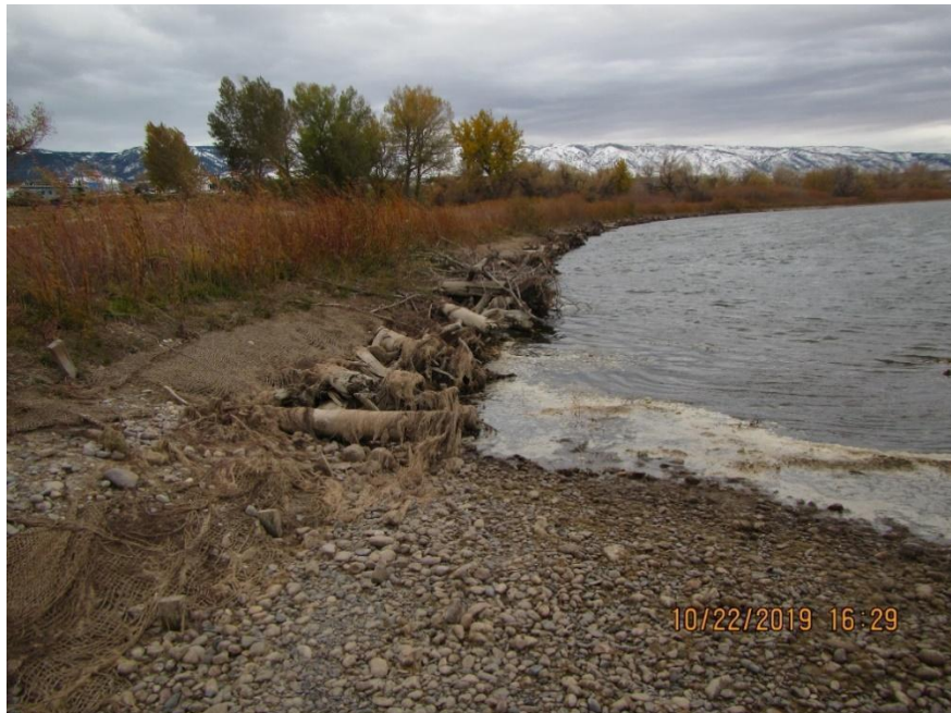
FIGURE A.5.2. Site 2 & 3 - Wyoming Blvd, standing at downstream end of toe wood 1, looking upstream. Willows have established well above the structure, contributing to long-term bank stability.
